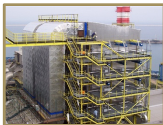
Brindisi Nord Plant
